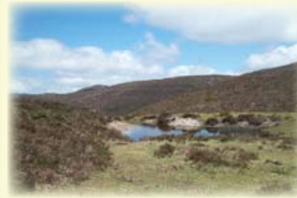
One of the reservoirs that provided the water needed for the Roman gold mines of the valley of Bustantigo.
